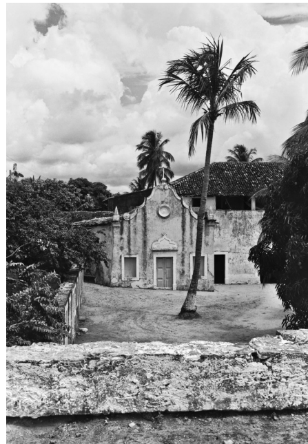
Chapel of the Fort Saint Ignatius, 1974 PHOTO: ALCIR LACERDA
